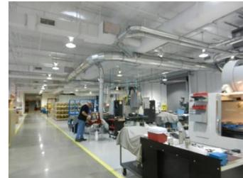
The flexibility was recently demonstrated in one of the campus warehouse locations when it was deemed that the air system needed to be raised to allow for higher stacking on the racks. Patton's were able to quickly address the issue and raise the system height, due to the flexibility of the wire hanging system.
