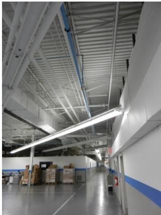
Because the production layouts are constantly changing (as often as every two weeks) in addition to over 3500ft of tubing, the 'Air Centers' team installed a large number of Infinity manifolds in the roof to allow for quick changes of production layout during weekend shutdown. This flexibility along with the worry free zero leak system has been a real benefit to the facilities team at Sparton.
